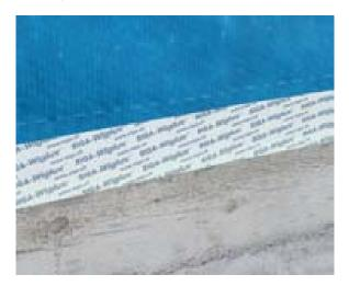
The base joint should now be sealed windtightly with SIGA Wigluv.
