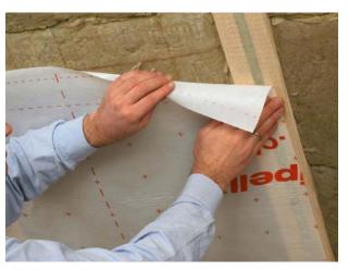
Fit SIGA Majpell with the slightly rougher fibre side towards the interior.
