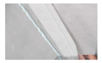
Apply 8mm bead of SIGA Primur and allow to rest for 1 to 3 days.
