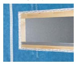
The window is sealed windtightly with SIGA Wigluv 60.
