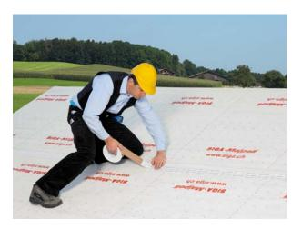
Bond overlaps and penetrations airtightly using SIGA Wigluv 60.
