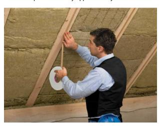
Use double-sides adhesive SIGA Twinet when mounting SIGA Majpell onto wooden substructures. Unroll SIGA Majpell and cut it to size.
