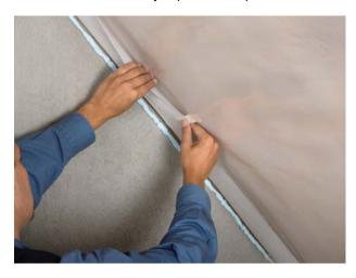
Release secured vapour control layer immediately after applying SIGA Primur bead.
