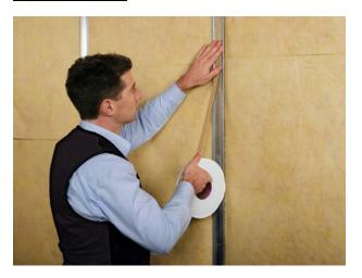
• Use double-sided adhesive SIGA Twinet when mounting SIGA Majpell on metal substructures
