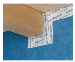
The angular penetration is sealed windtightly with SIGA Wigluv 60.
