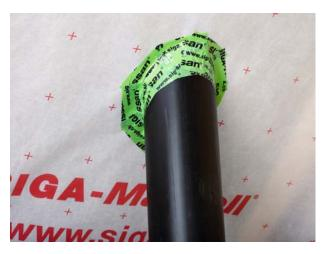
• The finished penetration should be durably and airtightly sealed with SIGA Rissan in layers.
