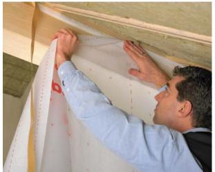
Bond vapour control layer to rafters with SIGA Twinet, or staple it on.
