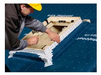
Seal the roof membrane all round the skylight frame so that it is windtight.
