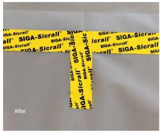
When airtight sealing a crease, a T-shape across the overlap should be used.
