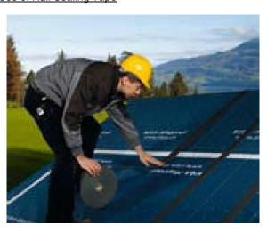
After sealing SIGA Majcoat roof underlay, bond the nail sealing tape to the underlay.
