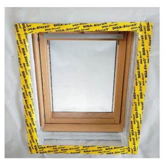
Airtightly seal vapour control layer sheeting overlaps with SIGA Sicrall.
