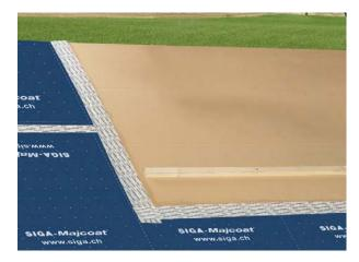
The transfer area between the covering membrane and the softboard is sealed windtightly with SIGA Wigluv and SIGA Dockskin.
