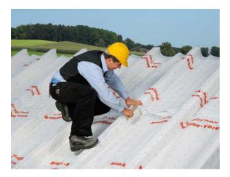
Bond overlaps and penetrations airtightly using SIGA Wigluv 60.
