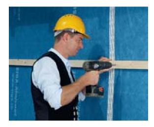
After adhesion, for final attachment of the membrane mount counter slatting in structure direction directly on the bearing structure.
